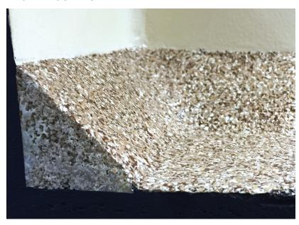
Note there is no 90 degree angle at the wall and floor, the "cove" at the juncture lets water flow away so there is less chance of bateria build up.
